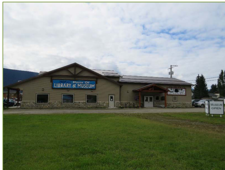
Robson Valley Exploration and Learning Service Building renovations in 2018.
