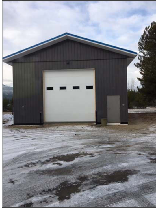
Valemount Fire Hall Garage Built in 2018
