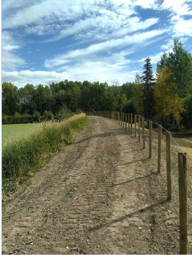
Tabor Lagoon Berm Repair
