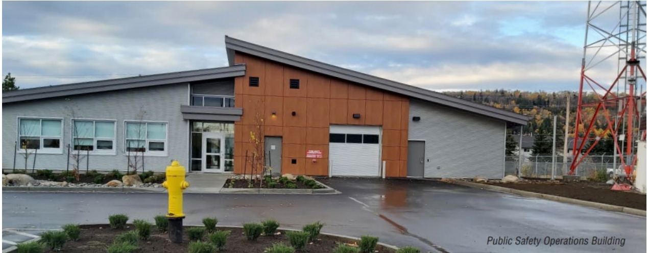
Public Safety Operations Building
