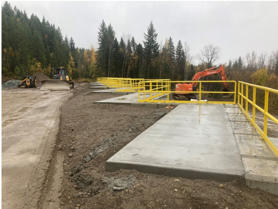
Cummings Road Regional Transfer Station Reconstruction
