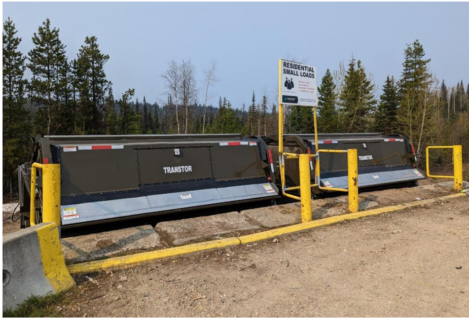
Bear Lake Transfer Station Bin Replacement
