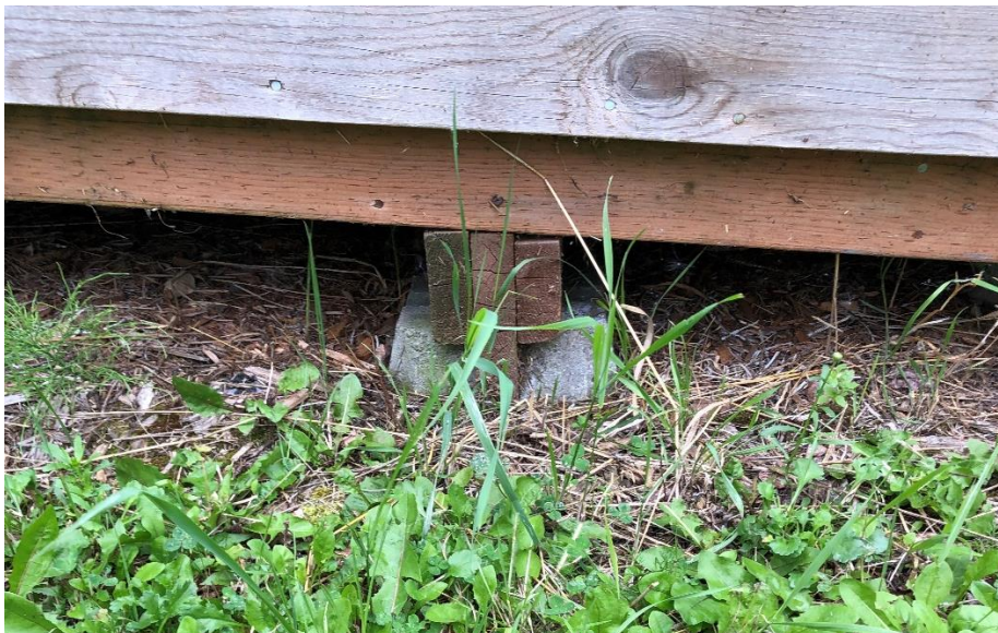
Photo 4: Wheelchair ramp supports
