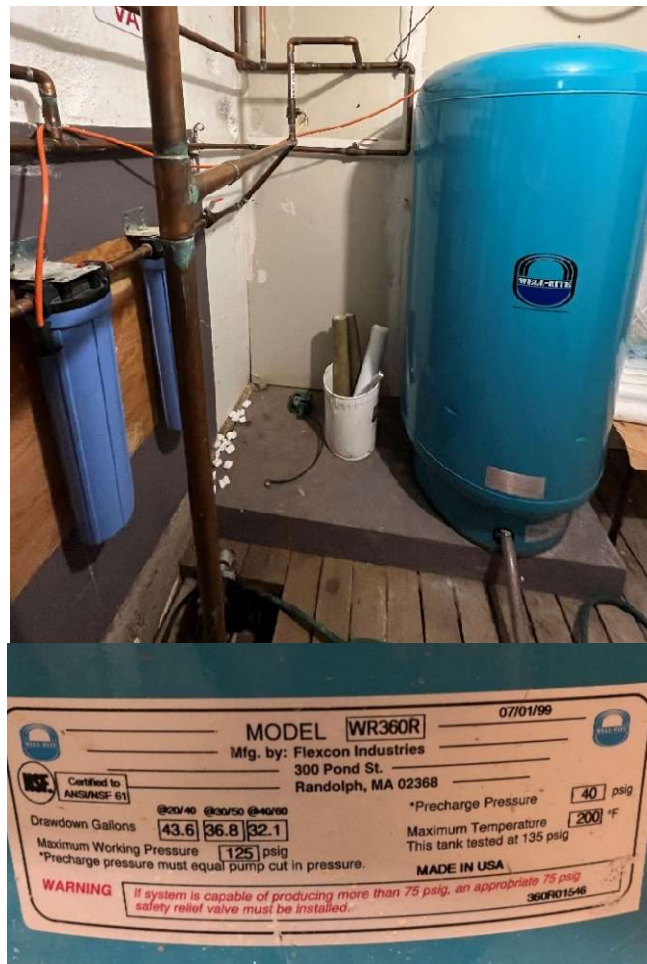
Figure 5: Existing Pressure Tank
