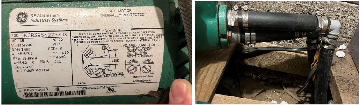
Figure 4: Existing Raw Water Pump and Motor Details
