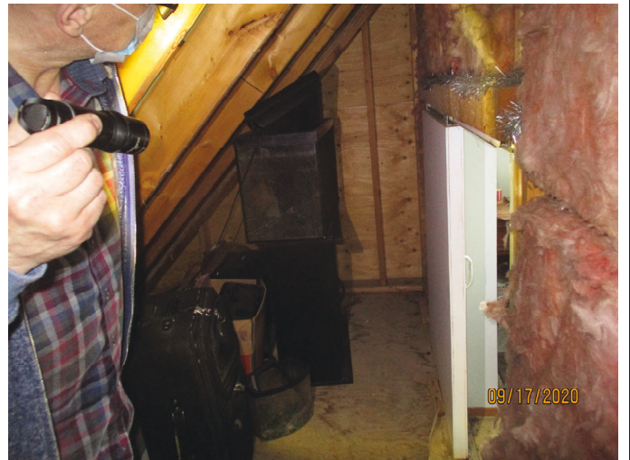
Photo 4: Shows hatch between north side attic and east side bedroom.
