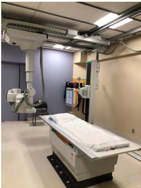
Mackenzie X-Ray Room Replacement
