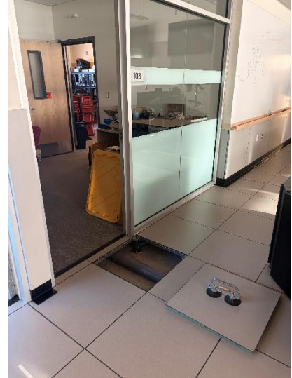
Figure 1 - Raised floor in front of Office 2 (Rm 108)
