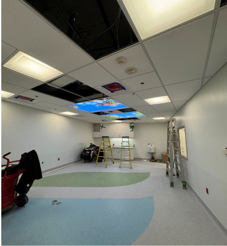
CT Suite Floor Finished and Therapy Lights Installed
