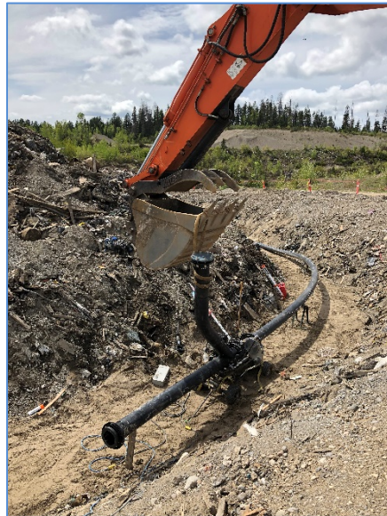
Landfill Gas Header Extension at Foothills Landfill
