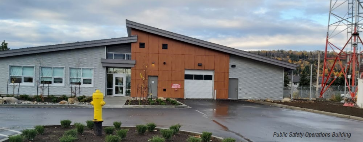
Public Safety Operations Building
