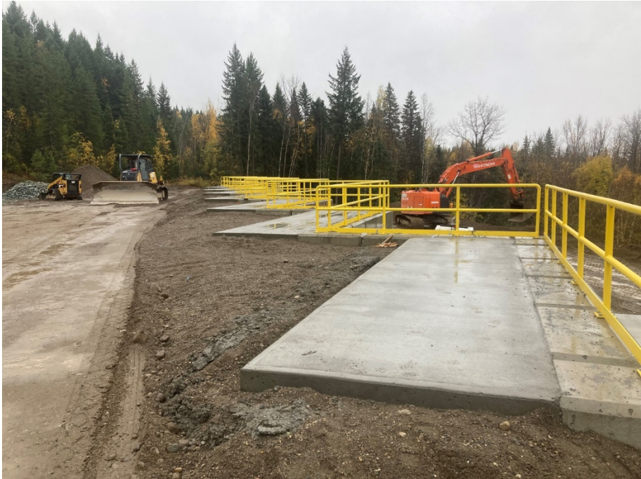
Cummings Road Regional Transfer Station Reconstruction
