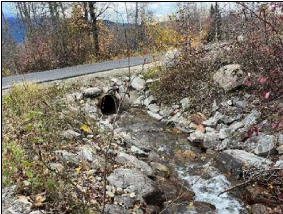
Photo 11: View of Rainbow Creek as it reaches Mountain View Road and passes under the road through a 1000 mm corrugated steel pipe culvert. Boulders are placed to armour the inlet.
