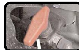
Manual Shutoff Valve
