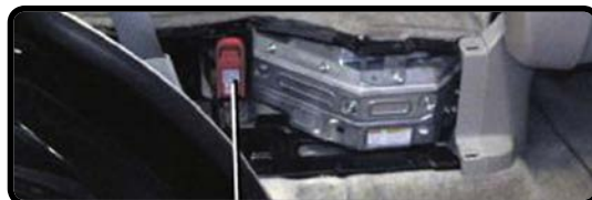
300V Hybrid Battery Manual Disconnect
