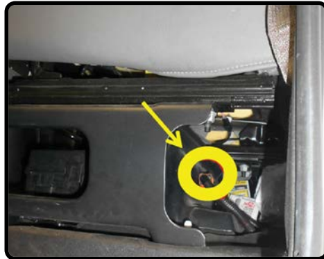
HV Disconnect Under Driver's Seat
