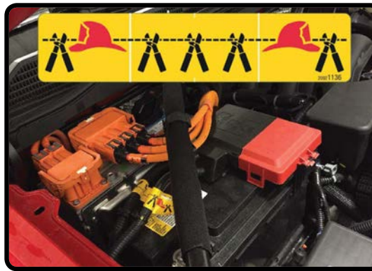
Cut All Marked Low Voltage Cables
