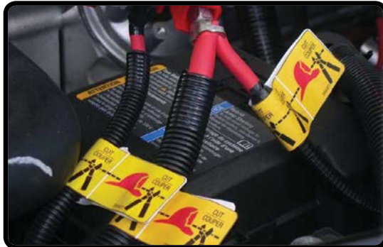
Cut 3 Exposed Cables (Alternate Procedure)
