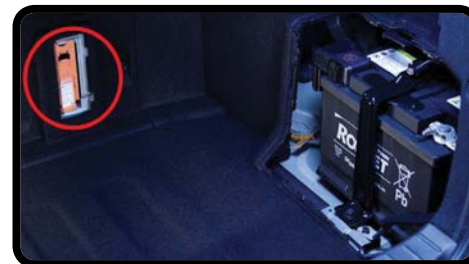
12V Battery and Service Plug in Trunk
