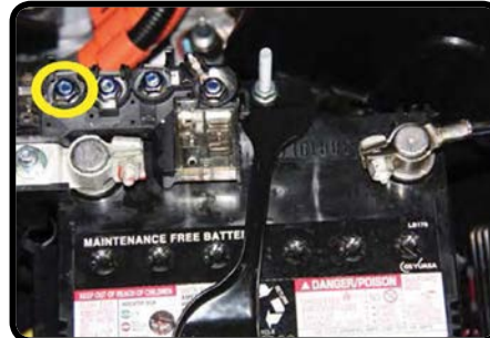
DC to DC Converter Connection
