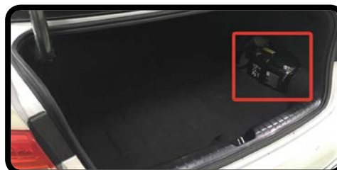
12V Battery Negative Cable in Trunk
