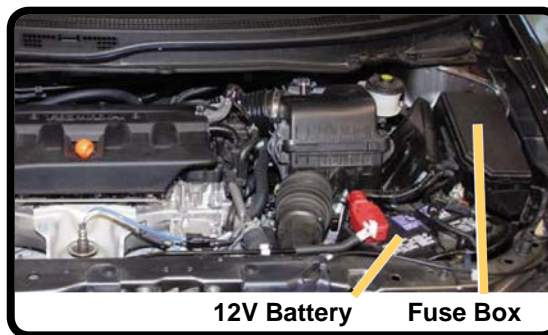
Fuse Box and 12V Battery Location
