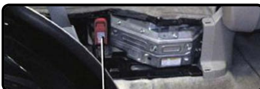
300V Hybrid Battery Manual Disconnect
