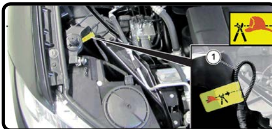
High Voltage Disconnect Under Hood
