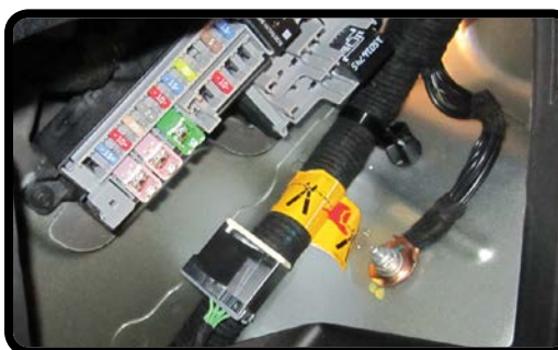
Cut through the positive 12V cable on each side of the tag to remove a section of the cable to ensure the cables cannot inadvertently reconnect.
