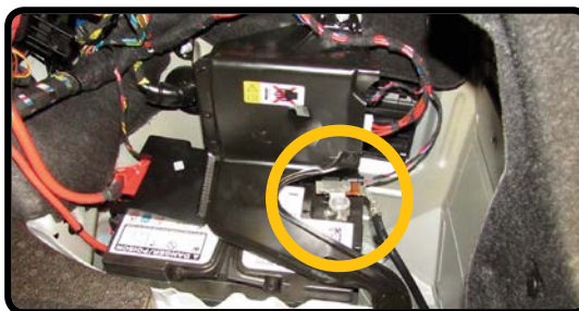
12V Battery Disconnect in Trunk
