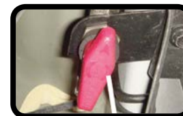
Manual Shutoff Valve
