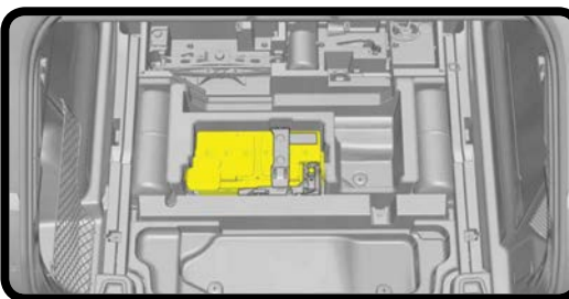
12V Battery in Trunk
