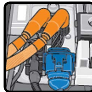
12V E-Box Disconnect
