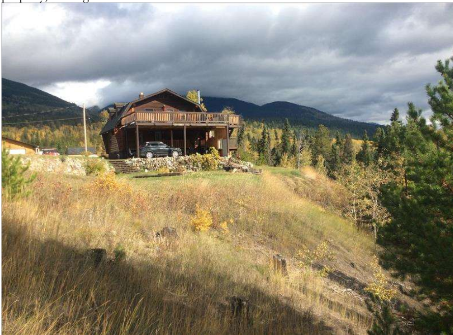
Photo 2 The rock armoured slope on the property and the existing residential structure setback from the escarpment slope, looking east.
