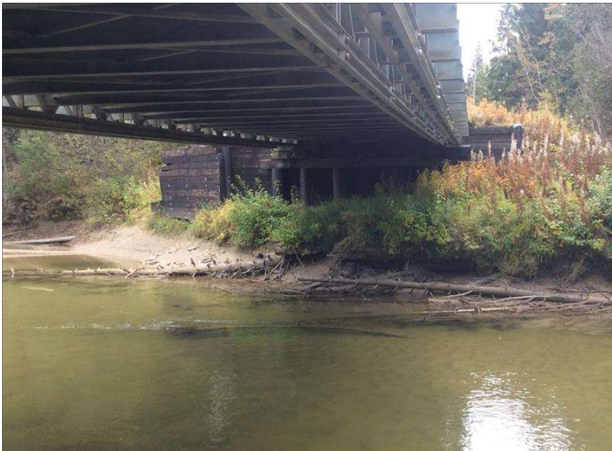
Photo 7 Bridge abutment at the crossing on Crooked Creek Road.
