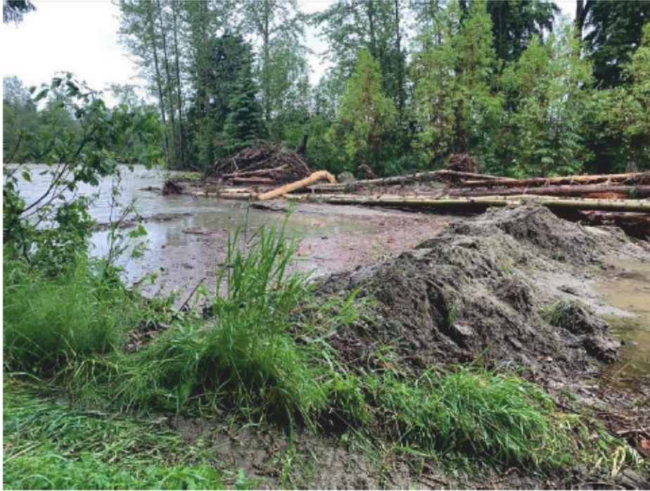
Photo 5: Berm constructed across low area by homeowner at 1655 Dorval Road
