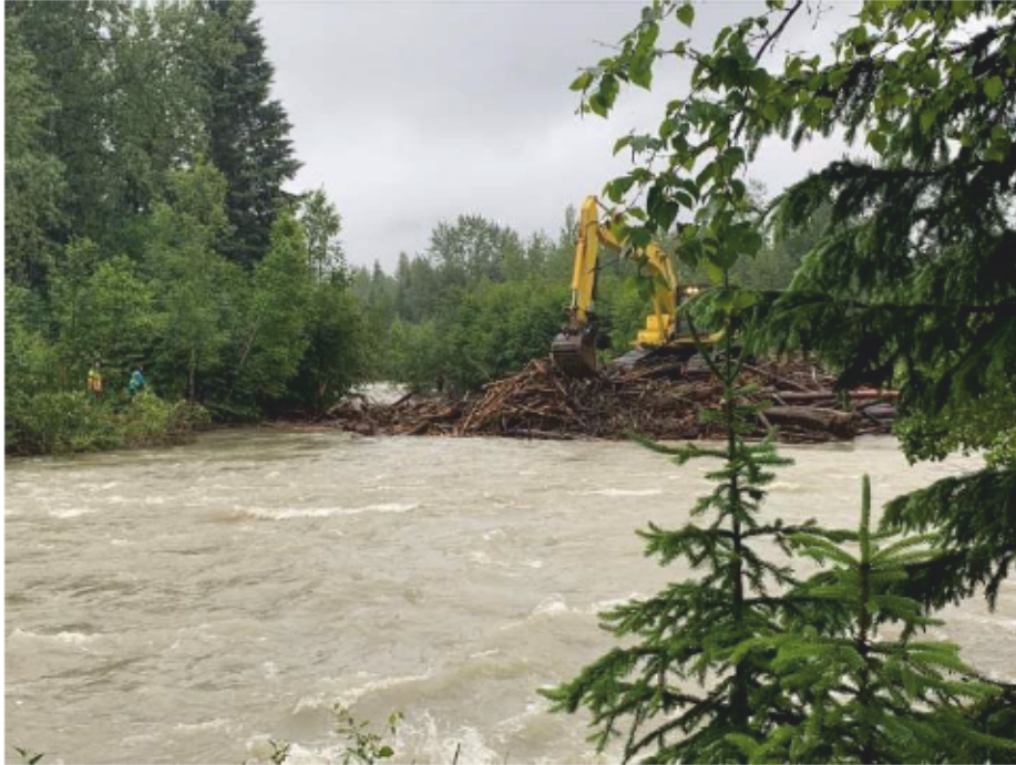
Photo 1: Excavator removing debris jam
