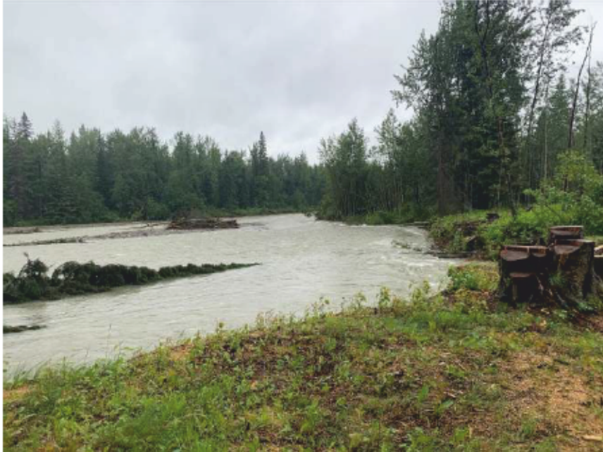
Photo 3: Looking downstream from the edge of the property located at 1005 Dorval Road. Property line use to extend out the gravel bar now in center of channel.
