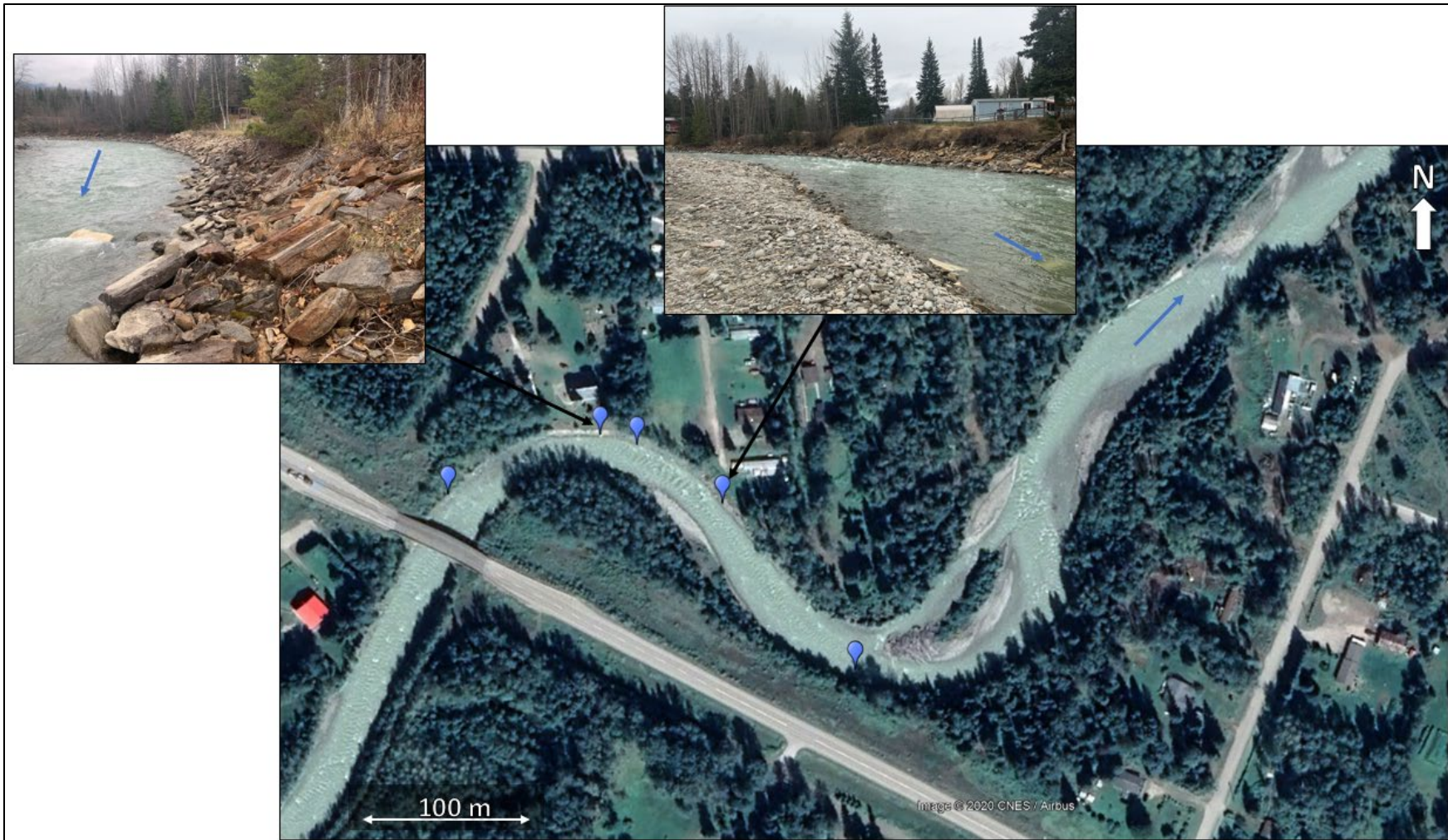
Figure 3-4. Riprap locations observed during a post-flood site visit by McElhanney are shown (blue markers) with flow direction indicated by the blue arrows. Imagery source: inset photographs obtained by McElhanney on November 3, 2020, and background imagery from Google Earth, August 19, 2019.
