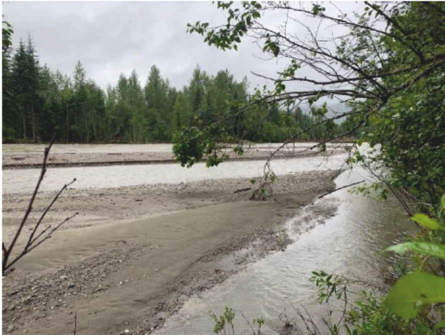
Photo 6: River channel and gravel bars in front of berm protecting community pumphouse
